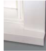
Historic designed sill nose, sloped to shed water
